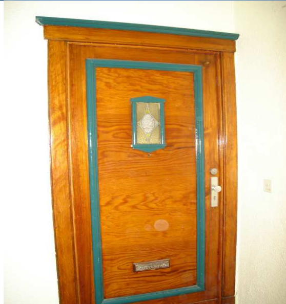
Door to the Apartment
